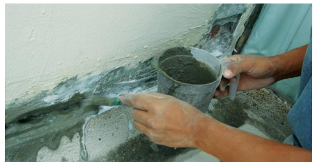
E P Bondex applied to crack before repair
